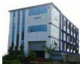
Tecnik Fluid Controls Pvt. Ltd. Mumbai, India
